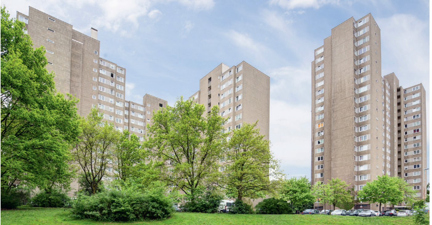
The 317 rental apartments are in high demand: Frankfurt is close by and the rents are attractive. Source: Capera
