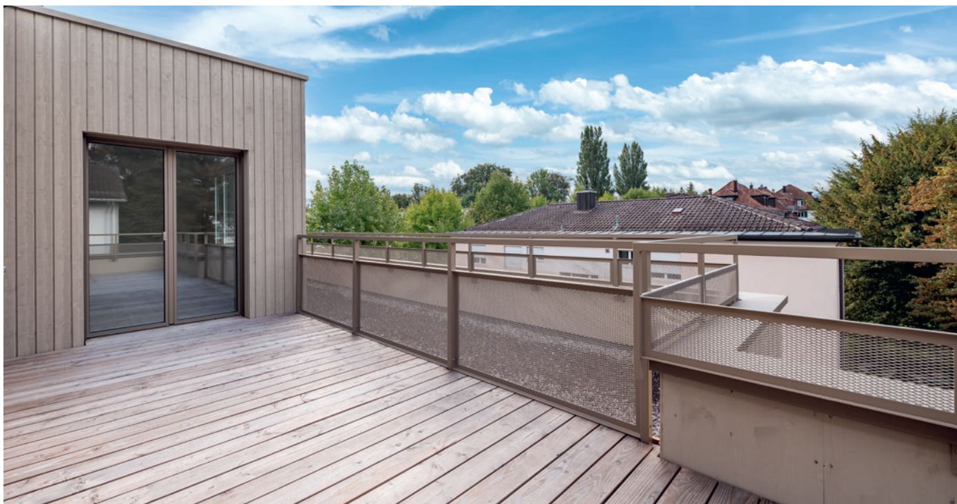
Generous use of wood creates a pleasant outdoor environment. Source: Fotowerder
