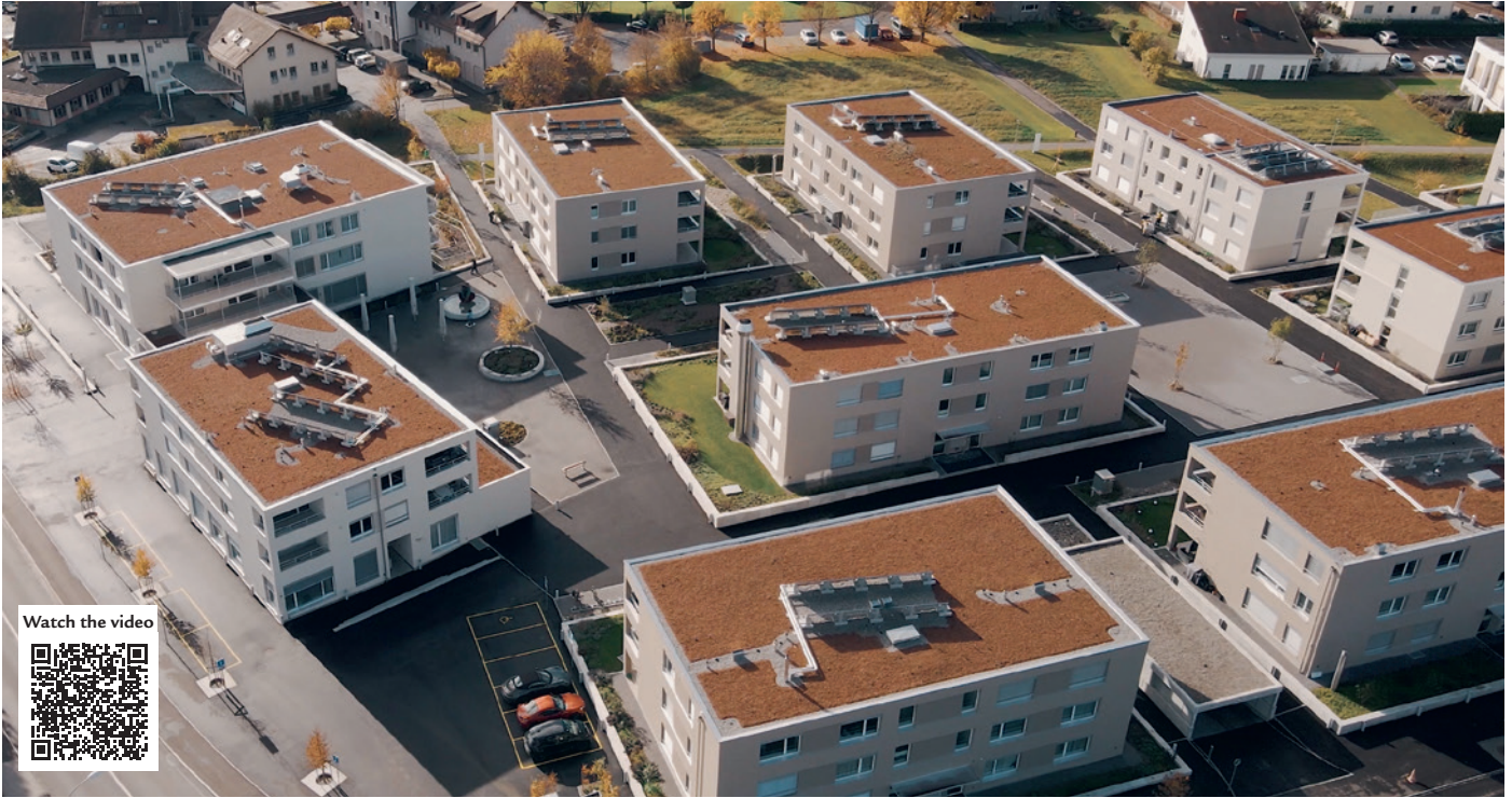
The complex received an award for its barrier-free accessibility. Source: Oase Service AG
