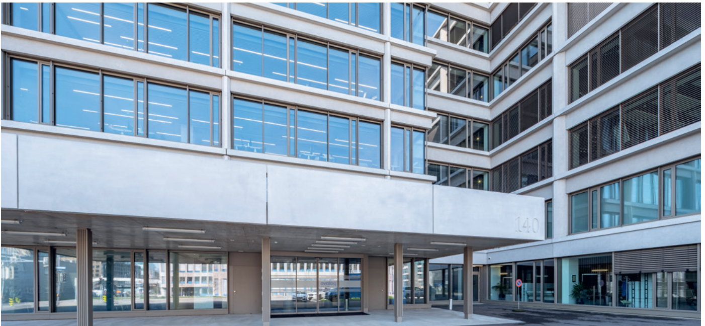
A base structure connects the two buildings on the ground floor. Source: Fotowerder
