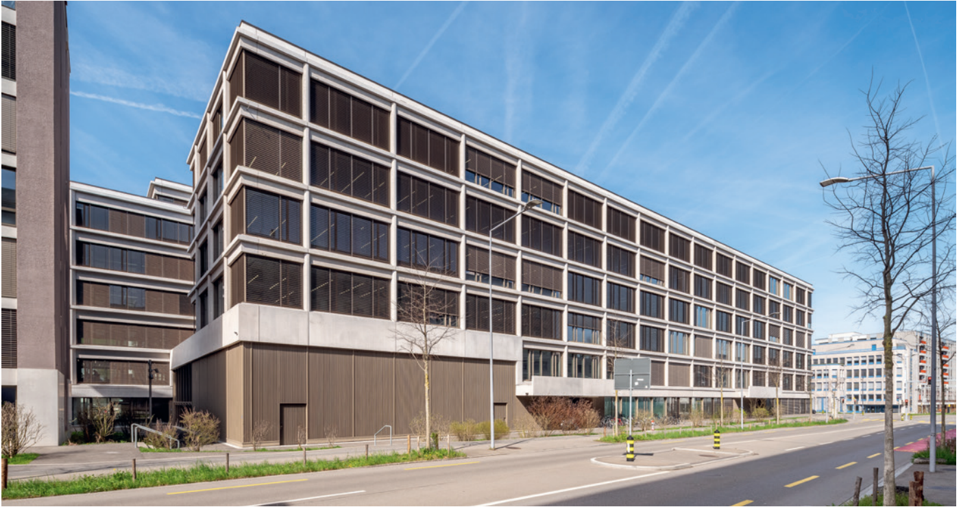
The high-quality, airtight building shell provides optimum heat protection in summer. Source: Fotowerder
