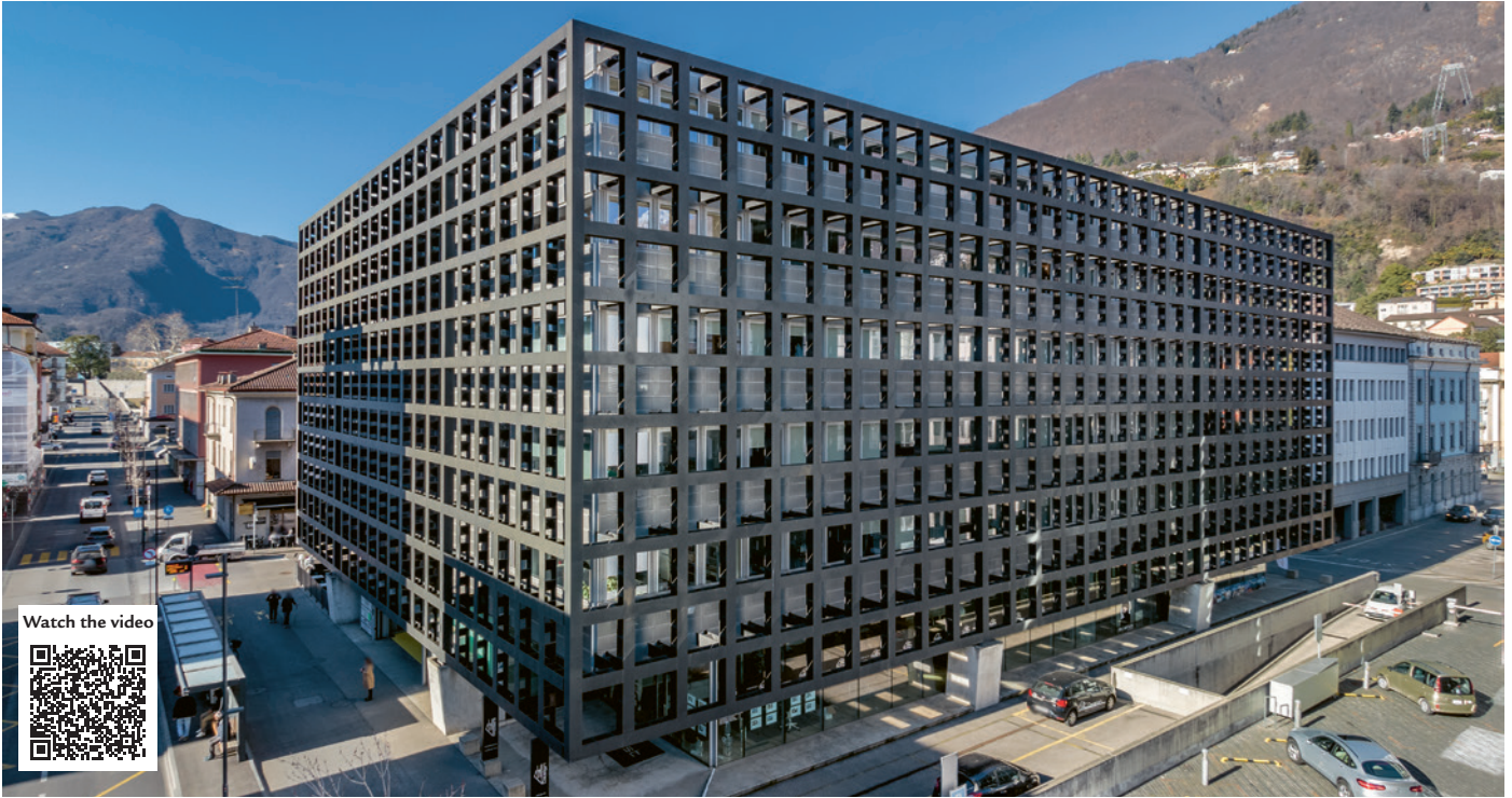
The striking architecture of “La Ferriera” – the “ironworks” – is unmistakable. Source: Fotowerder
