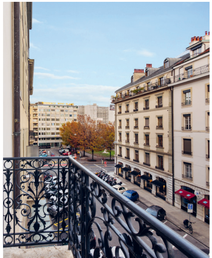
Iron railings are typical of the construction year 1893. Source: Backbone
