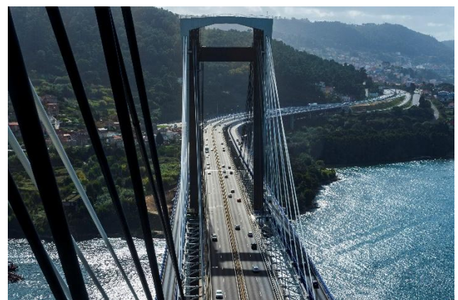
Rande Bridge, Motorway AP-9. Source: Punto GA, M. Riopa
