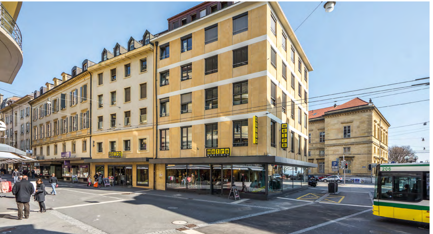
Corner location with excellent visibility. (Photo: JLL)
